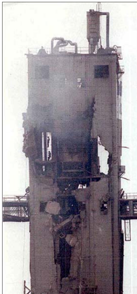
Figure 2. Destruction resulting from a combustible dust explosion at the DeBruce Grain Elevator 2
